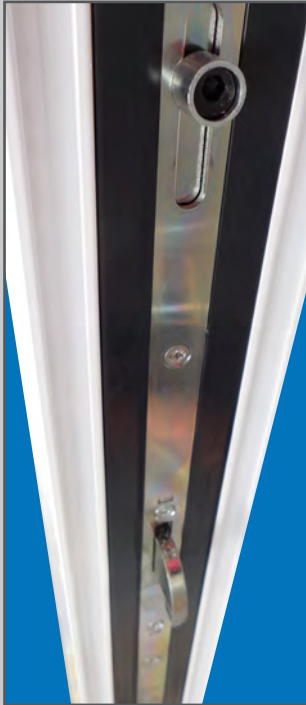
View of lower hook bolt and cam
